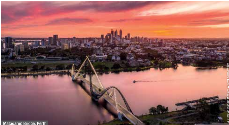
Matagarup Bridge, Perth
